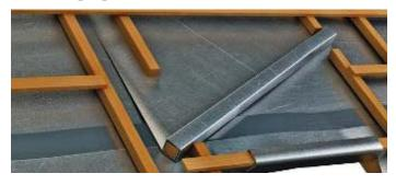
A strip of **SKYTECH PRO XL** external facing carefully separated from the rest of the underlay and whose width equals the distance between the rafters increased by 20cm must be cut up.
