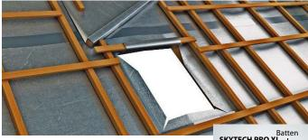
✓ Make 10cm to 20cm strips and fix them on the counter-battens around the header.
